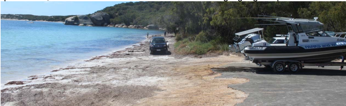
Figure 7.5 Two Peoples Bay Boat Ramp – Note Steep Drop-off
